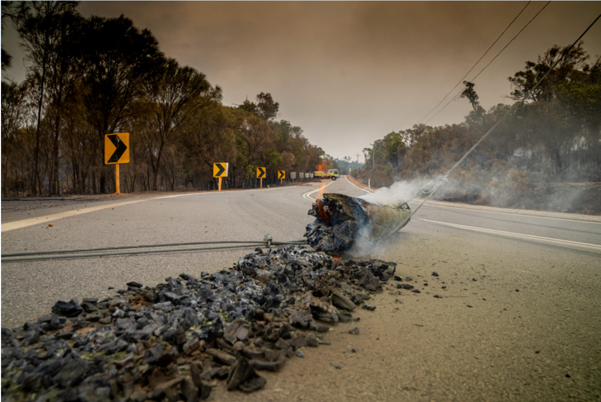
Image: DFES Incident Photographer Evan Collis
